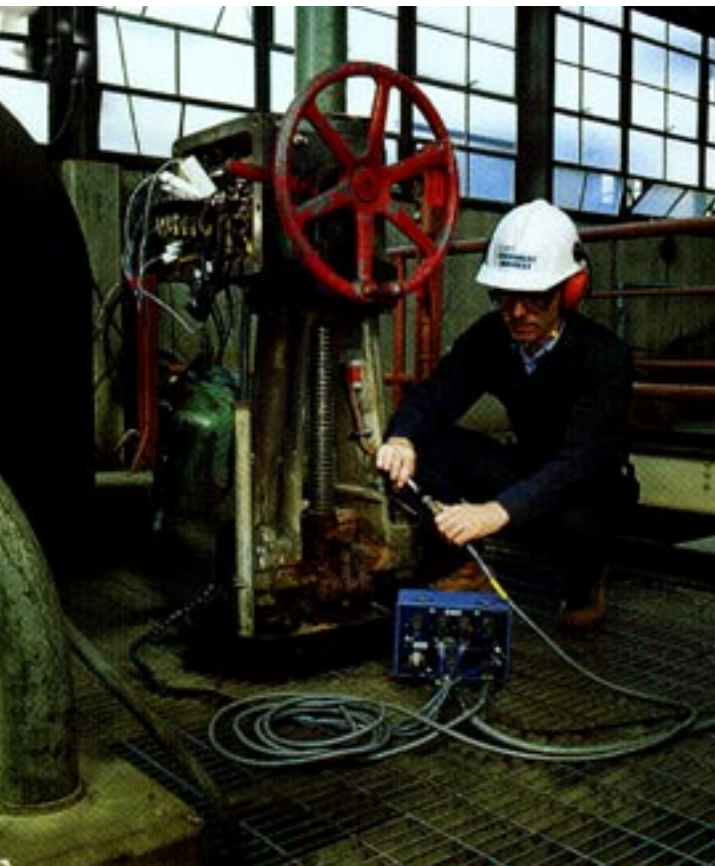
Developments in valve condition monitoring and testing continue apace with innovations coming largely from the nuclear power industry. Photo courtesy of Liberty Technologies Inc.
