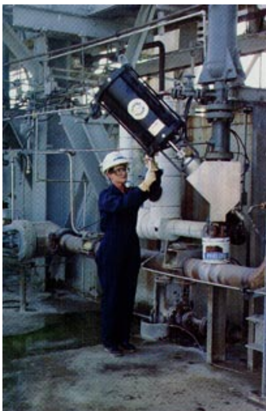
Y-conduit valves provide soft-seat, bubble-tight shutoff at pressures to 8,000 psi in fire protection vent application.
